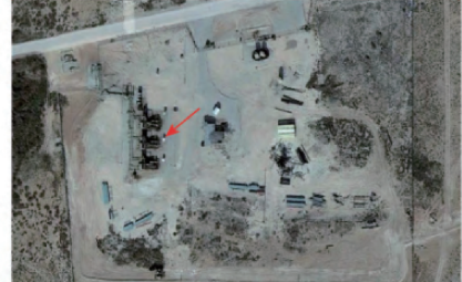
(b) 新墨西哥州埃迪县 Matador 压缩机组 (b) Matador compressor station in Eddy County, New Mexico
