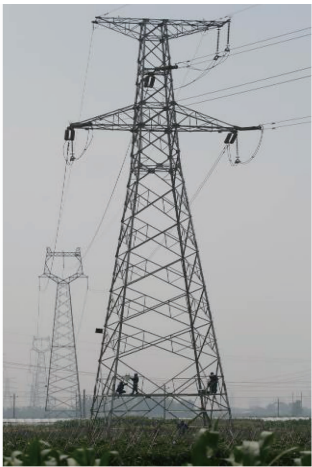
(a) 实验耐张转角塔 (a) Experiment tension resistance angle tower
